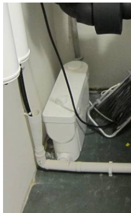
Figure 20: Pump removing overspill from DI water unit to drain.
