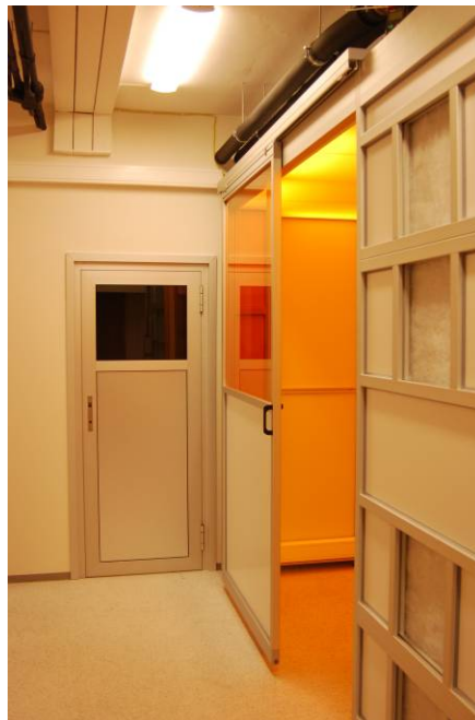
Figure 24: MCRT-cabin with sliding door entrance to e-Line. Squared air-inlets with filter fabric can be seen on the right. Cooling water supply can be seen on the top.
