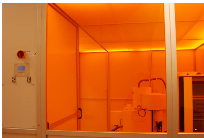
Figure 25: View into cabin from operator terminal.
